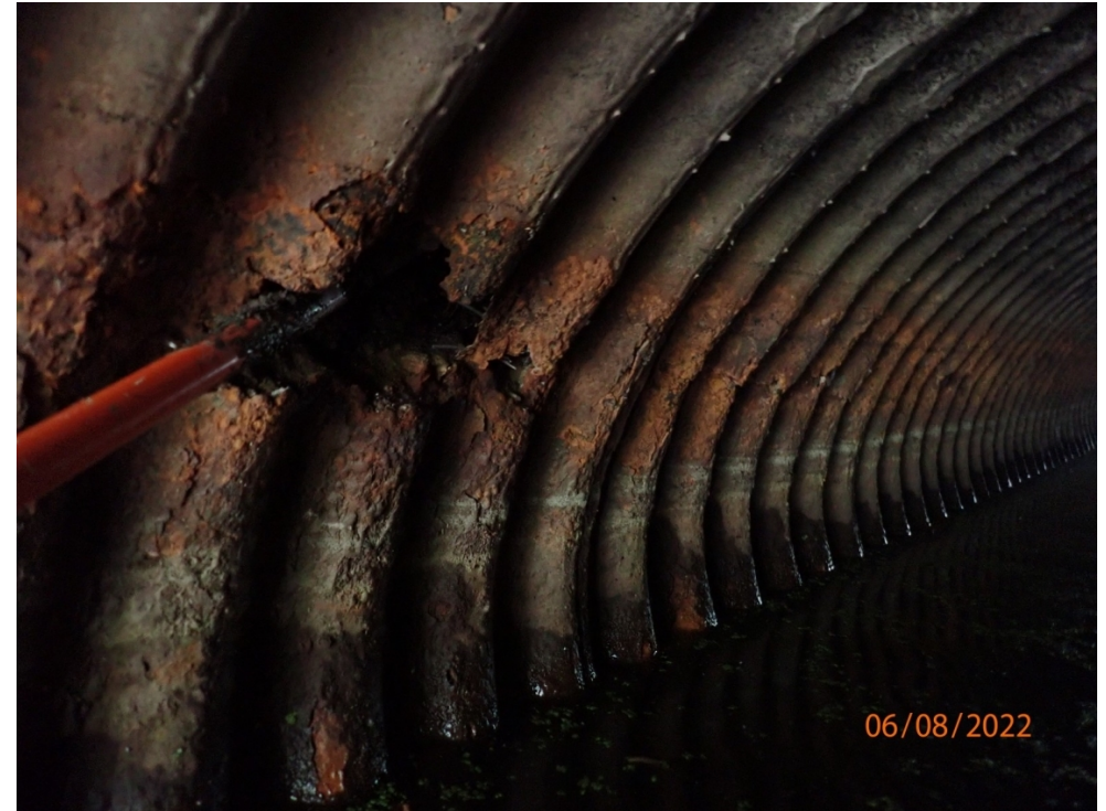
Section loss of the pipe creating a void where material has entered the pipe.
