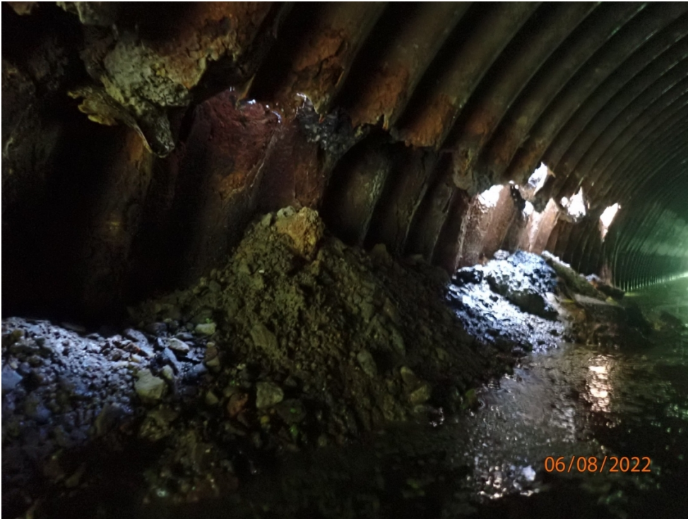
Daylight entering the pipe from the cave-in above located within the roadway surface.
