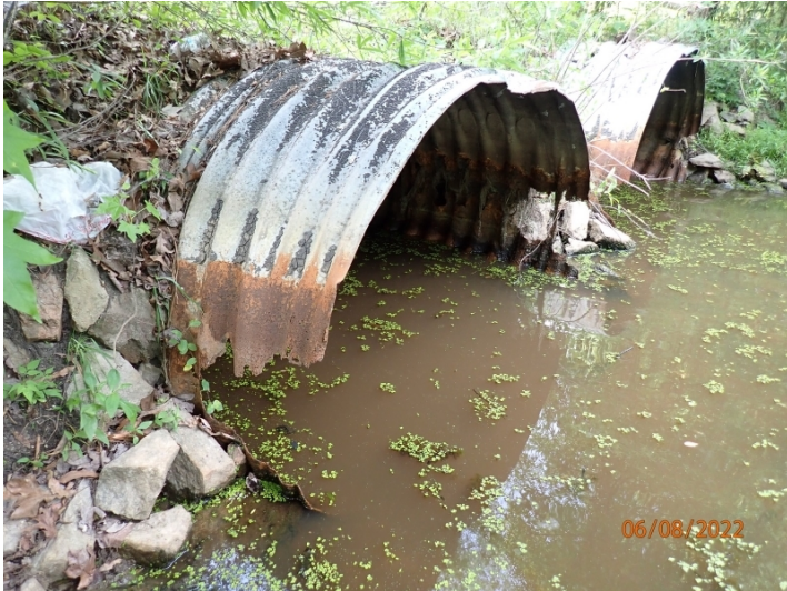
End of cross pipes showing section loss at the median flow line of the pipes.
