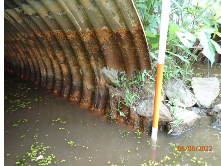
End of cross pipes showing section loss at the median flow line of the pipes.
