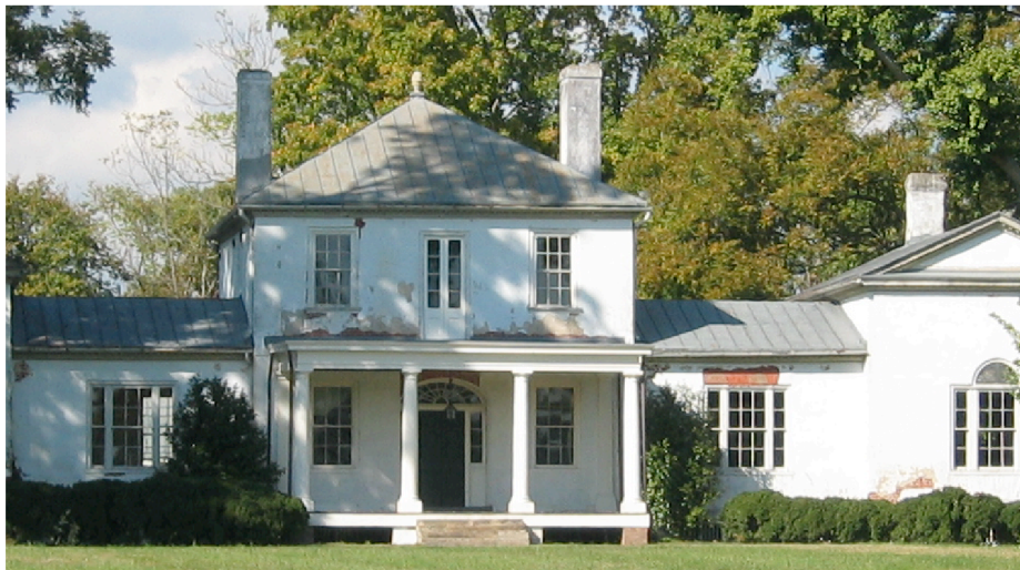
Battersea’s central building exhibits a hipped roof, hyphens are side-gabled and wings end-gabled. All are clad in standing-seam metal.
