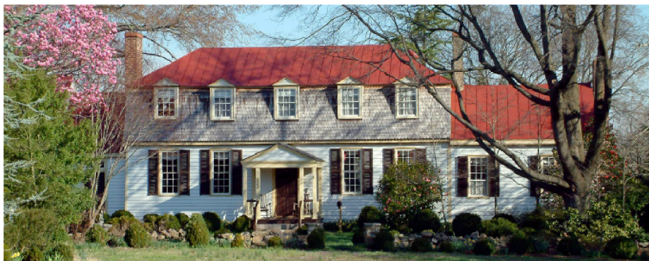
An early gambrel roof is covered in a combination of wood shingles and standing-seam metal.
